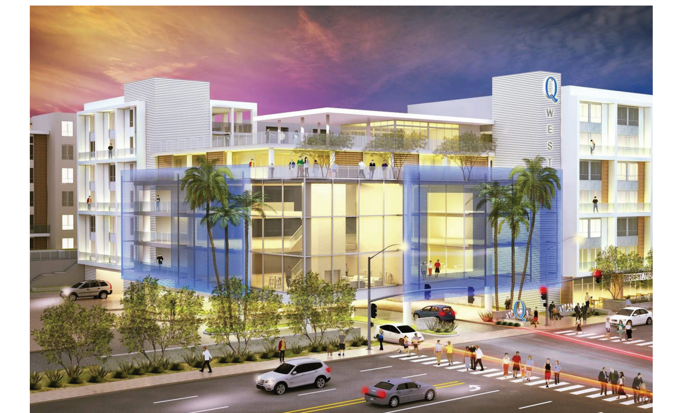
6 6263 Topanga Canyon Boulevard
